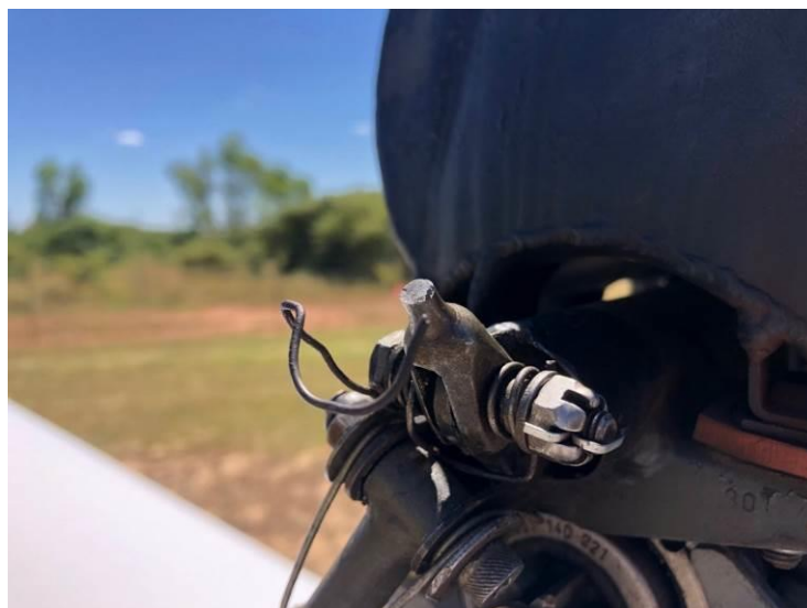
Figure 8: Broken Turnbuckle Near Head of Engine Pylon
